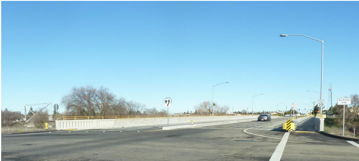
Pioneer Bluff Bridge
