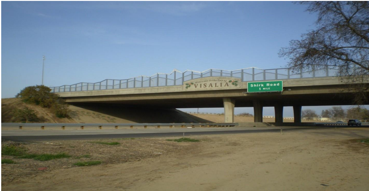
Visalia Bridge Airport Drive and SR 198 Source: City of Visalia
